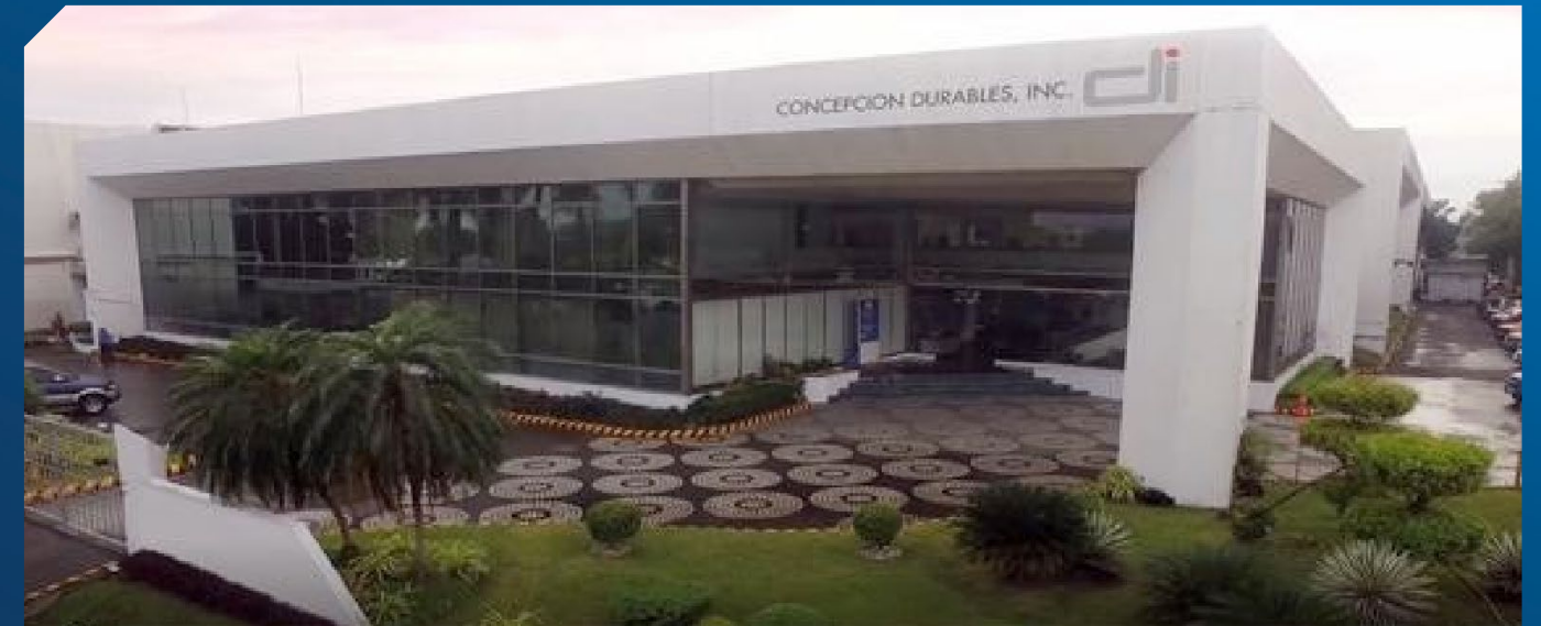
CDI Refrigeration Manufacturing Plant
